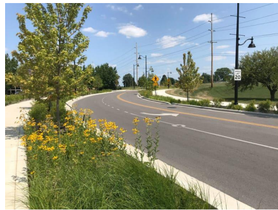
Bioswale green stormwater infrastructure.
