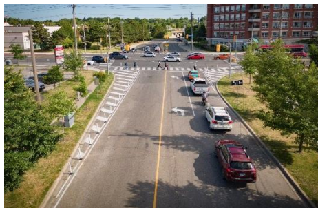
Reduced curb radii speed management.
