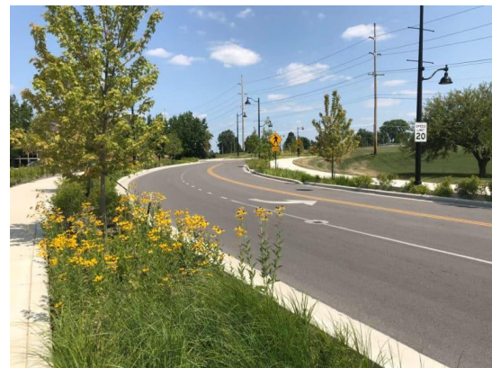
Bioswale green stormwater infrastructure.
